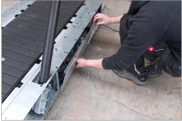
Fig. 42 Mercury/Path assembly, electronic cover plate
